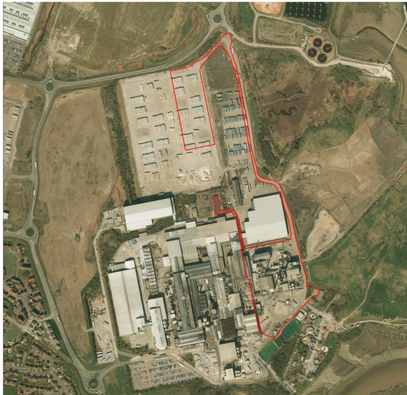
Figure 3.1 – DCO Boundary overlaid on aerial view of proposal site (K3 development not shown)
